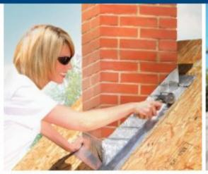
Peel & Seal<sup>®</sup> is an ideal choice as a flashing material around chimneys, roof vents, stack pipes and other difficult to waterproof items. Peel & Seal<sup>®</sup> can also be used to completely cover, flash seams or repair metal roofing systems.
